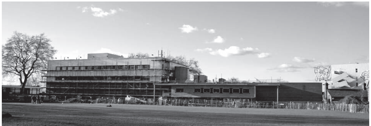
Right: The new Whitehead Building exterior is being revealed.
