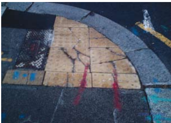
A participant's photo of an example of poor urban design: it is very easy to trip because of uneven pavement
