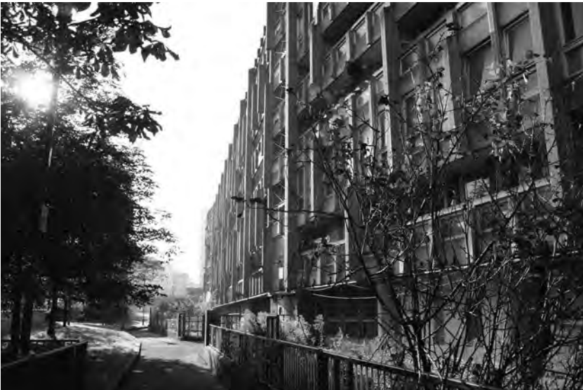
Figure 6.7 Mullions as sun-responsive forms, on the west-block garden façade. (Nicholas Thornburn, October 2015)
