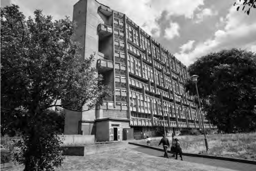
Figure 1.3 Robin Hood Gardens, garden façade of the ten-storey east block. (Kois Miah, June 2015)
