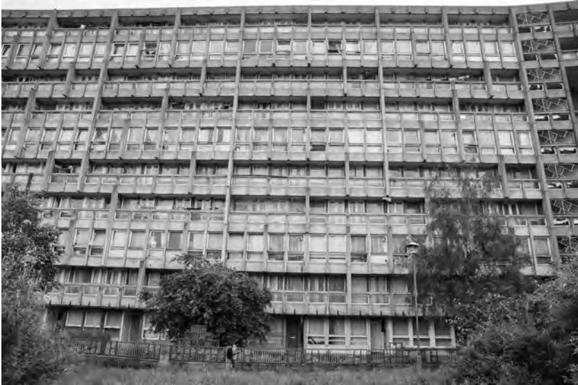
Figure 6.5 Garden-facing façade of the east block. (Kois Miah, May 2016)
