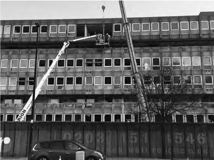
Figure 8.4 Dismantling housing for heritage at Robin Hood Gardens. (Nicholas Thoburn, 2018)
