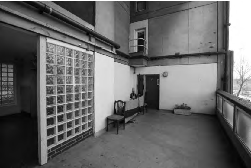
Figure 3.9 A west-block head maisonette and triple-height street deck, with lift-lobby to the left. (Kois Miah, April 2015)
