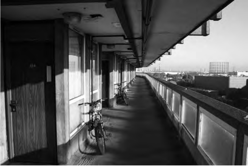
Figure 3.2 Street in the sky, east block, looking north. (Nicholas Thoburn, February 2015)
