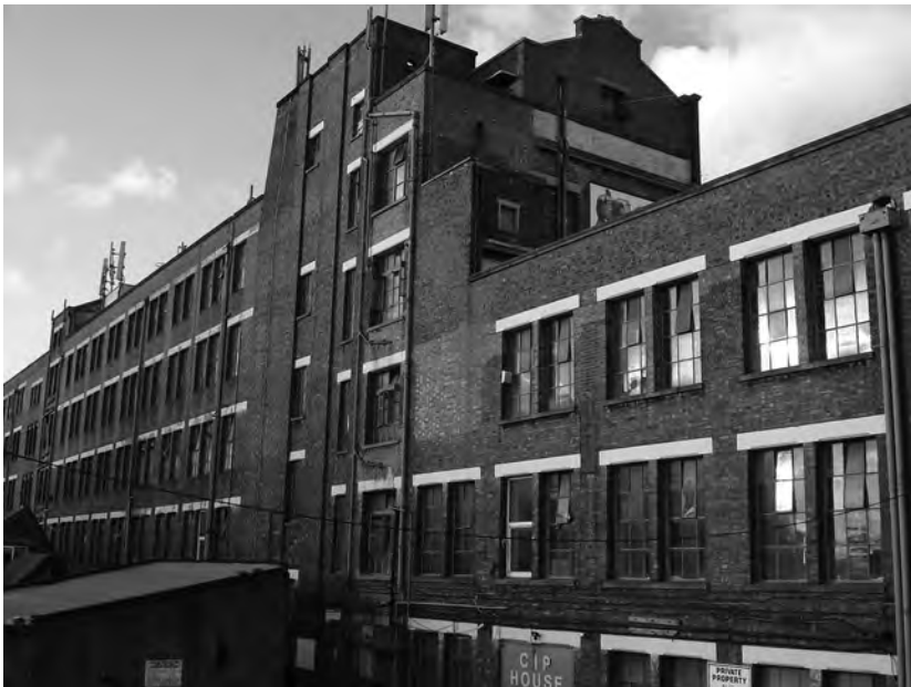
Figure 8.5 The Bussey Building before conversion (image credit: courtesy Benedict O’Looney Architects).
