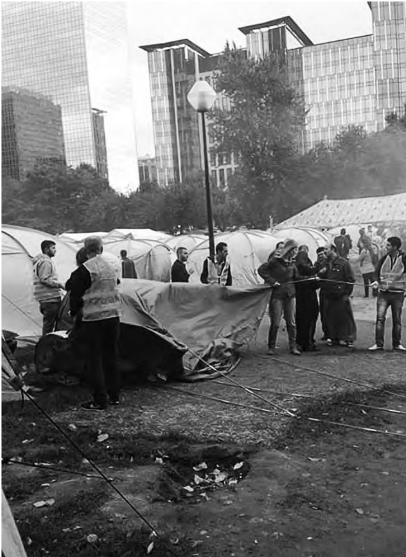
Figure 6.20 Brussels, Belgium, 2015. Volunteers erect a tent that will be the first school in Parc Maximilien.
